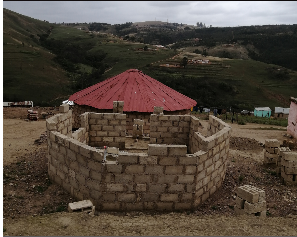
The building work taking place
