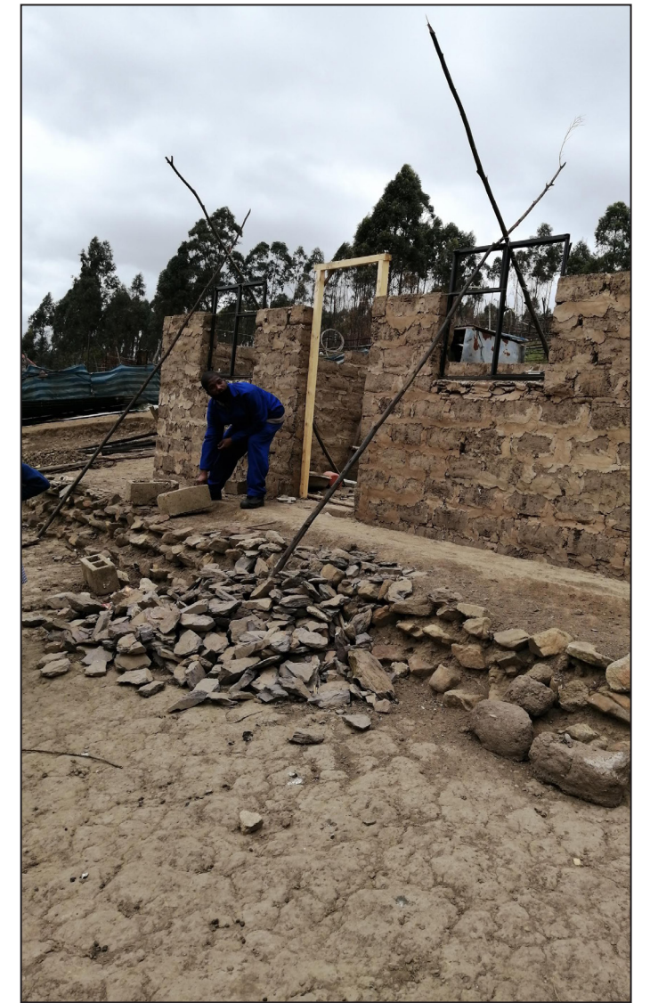
The building work takes place
